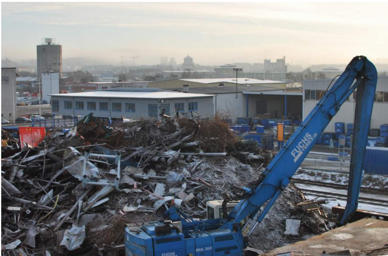
Figure 30. Mixed steel waste is being sorted and shredded
