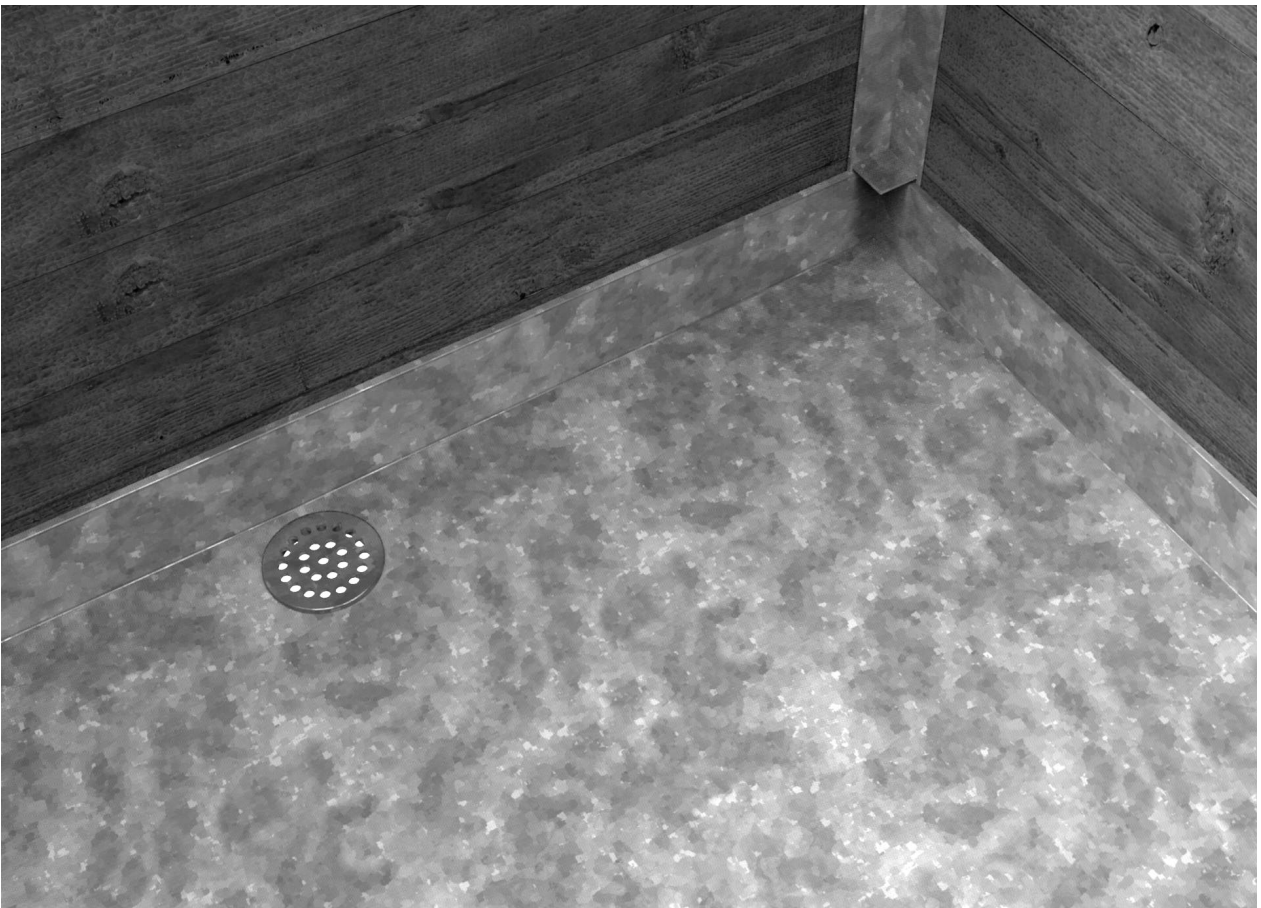
Figure 37. Grid and bottom plate with drainage hole.
